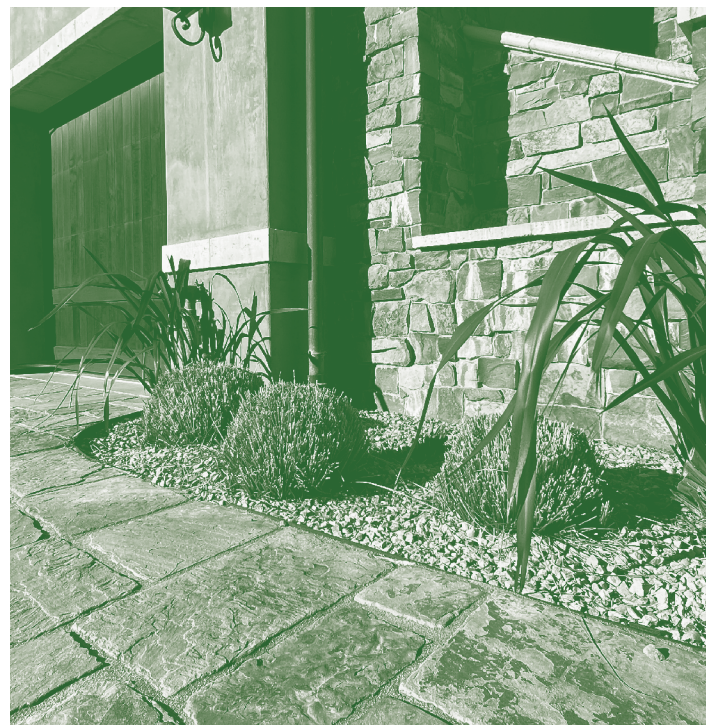
Landscaping requirements that address areas within five feet of a home help reduce ember ignitions. Image: Napa County Fire Department
